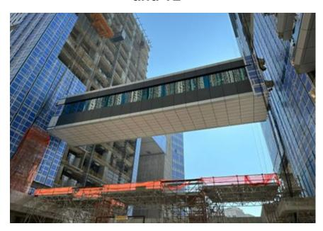
In February 2022 Harmony Construction Co. Limited were awarded the Contract for the design, supply and operation of heavy lifting operations on a steel truss link bridge at the HK Immigration Headquarters. The works were conducted at Area 67 TKO between buildings T1 and T2. The link bridge had a total weight of 380 Tonnes.
